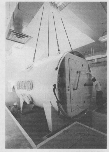
WORKERS lowered one of two 33-ton walk-in blast chambers through the roof of an ECF firing bay recently in preparation for the building's opening. Roy Dickey, a contractor in Explosive Projects & Diagnostics Dept. 2554, designed the 19-ft.-long, 11-ft.-diameter chamber, inside which up to a kilogram of explosive material can be detonated. Each chamber comprises some 2,000 parts, including mechanical, electronic, and optical components.
